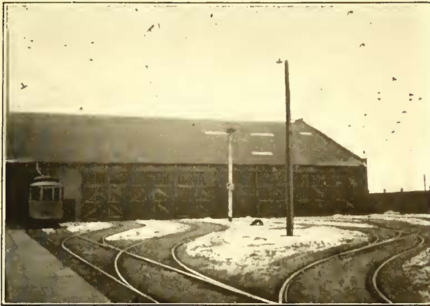
ENTRANCE TO INSPECTION SHOP OVER NEW TRACK LAYOUT
