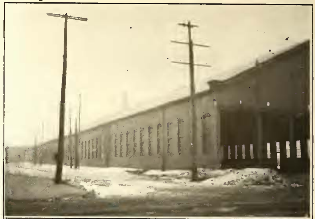
SIDE AND ENTRANCE TO CARHOUSE FROM CLEVELAND AVENUE
